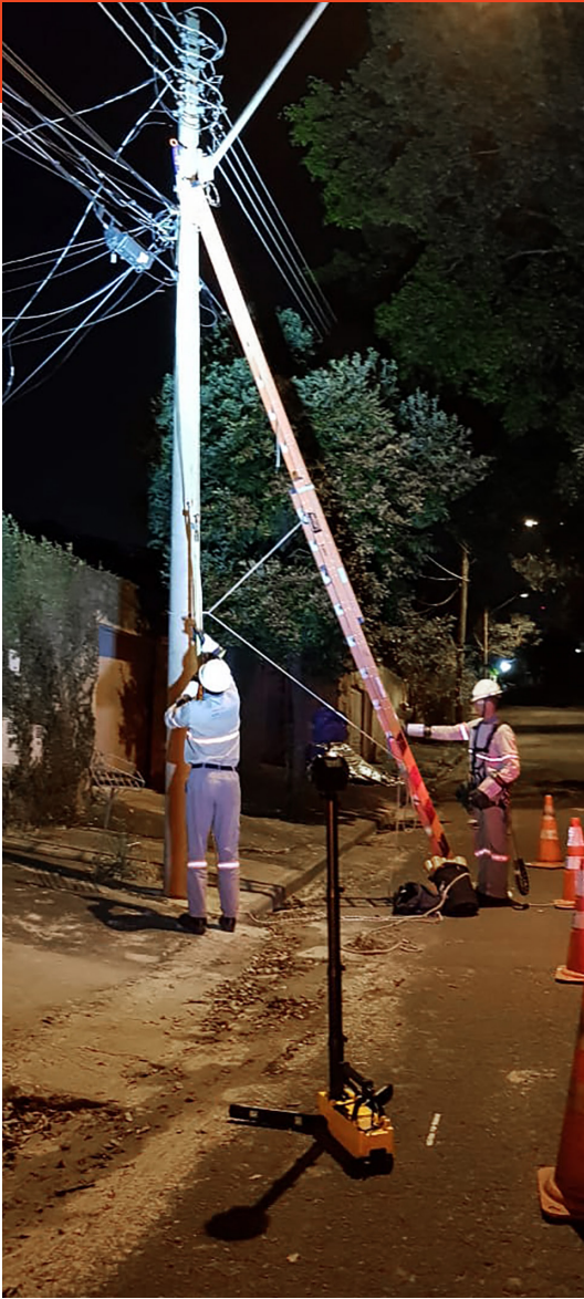
Extends to full height with the stabilization legs fully deployed and locked in less than 30 seconds
